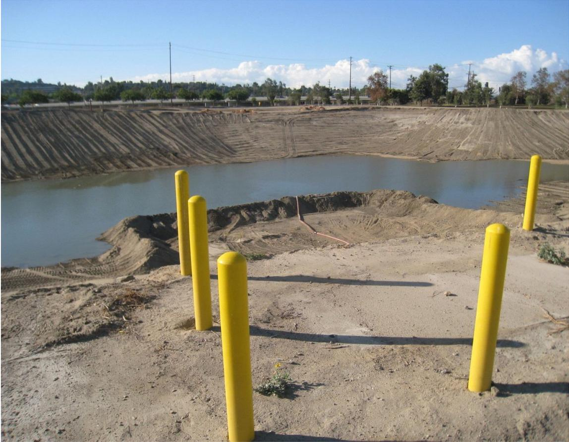
Here are the yellow barrier pipes that mark the location of the new 8 foot pipe between the Trout Lake and Chris's Pond. The big pipe is 20 yards to the right.
