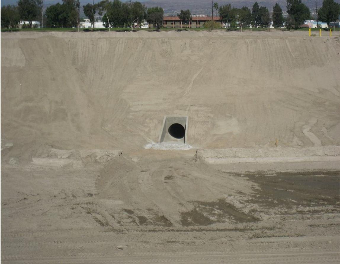
The “Three Pipes” are gone. The rusted out pipes were removed and this giant 8 foot tall pipe was installed at the bottom of Chris’ Pond. This is an important modification; it allows the circulation of water at the bottom of the Lakes, increasing water quality.
