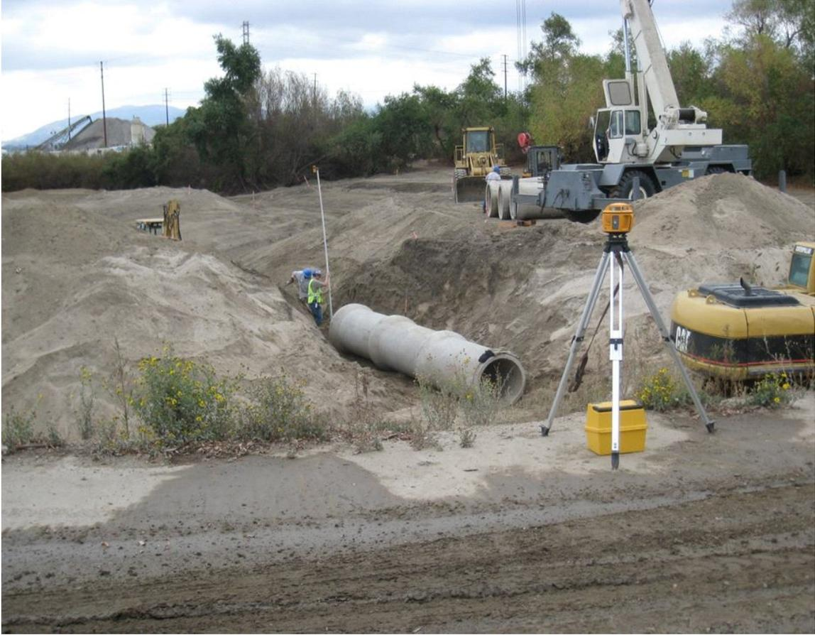
Installing the new pipe from “Trout Channel” to the main channel feeding the Bubble Hole in the Trout Lake.
