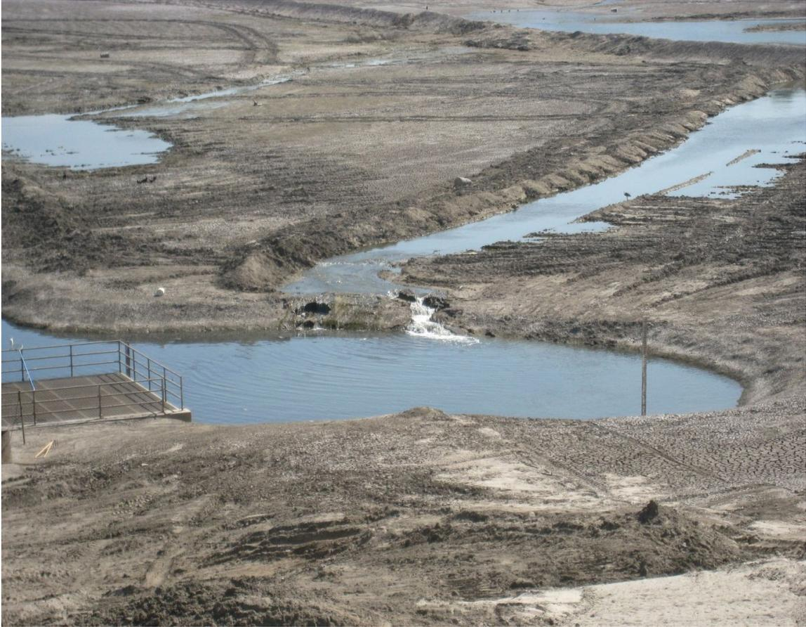
Note the Trout Lake is completely drained. But because of the fresh water pouring into the Lake from springs, this water had to be continuously pumped out of the Lake so that the big main pumps, inside the concrete structure to the left, could be removed and repaired. Note the volume of water filling the areas to the right and the channel.
