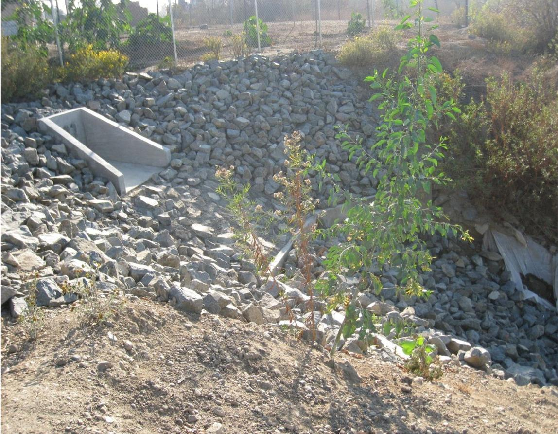
Great rocky structure below the pump station in the South East end of the Catfish Lake, left of the spillway.
